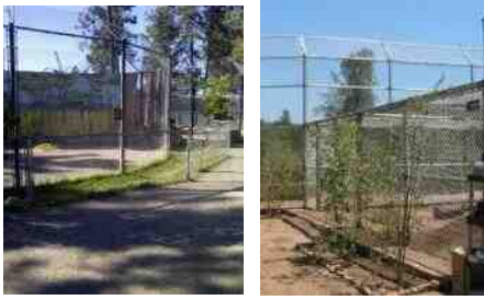
Compliant big cat fencing
