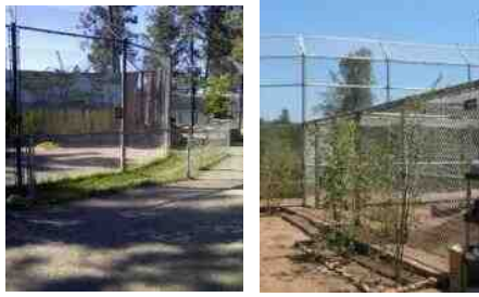
Compliant big cat fencing
